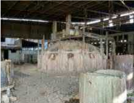
Figure 5: Pot Furnace - Sample Photograph
