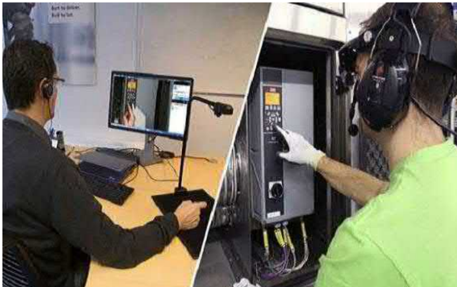
Fig 12. Remote maintenance using AR (Thanks to Gabler)
