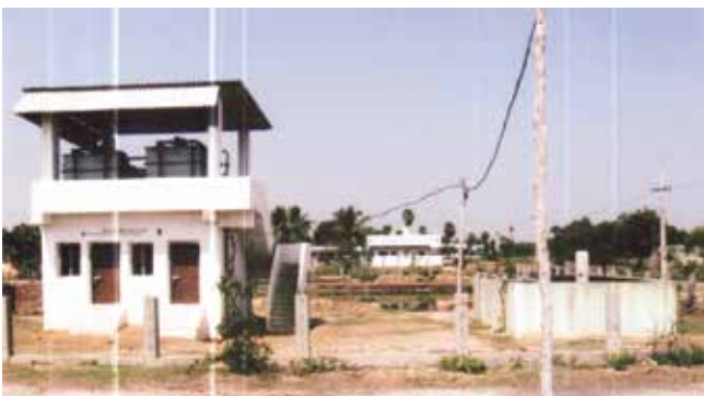
Common Effluent Treatment Plant
